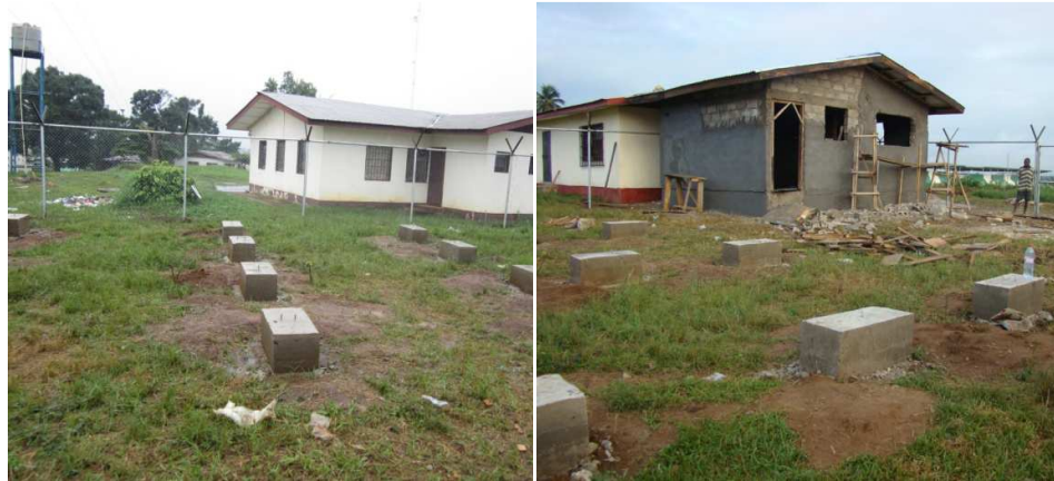
Figure 15 - Ganta 15 kW PV system in construction (MYS building on left and battery house on right)
