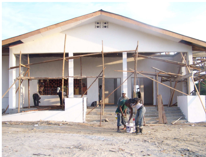
Figure 6 - Construction of RSTI in Harper ongoing in August 2012
