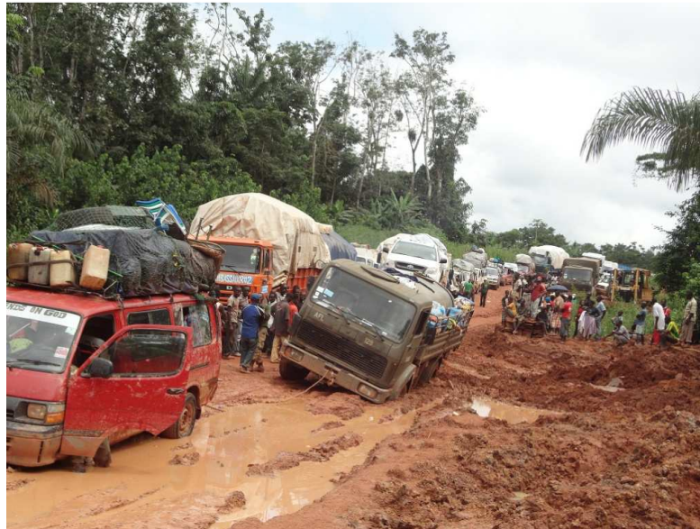
Figure 9 - Typical road conditions in the east of Liberia
